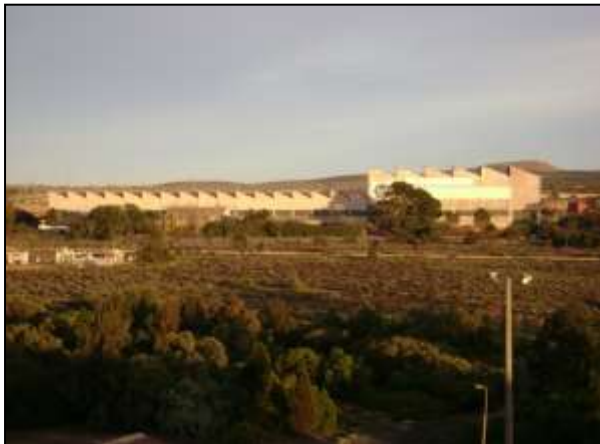
E&A Building – Whyalla S.A.
