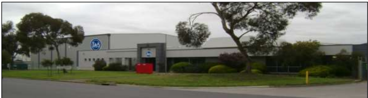
Engineering and Services Centre – Wingfield SA.
